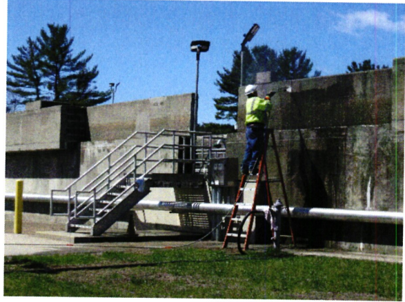
Seasonal power washing of concrete at Veolia's Southbridge, MA, WWTP Project
